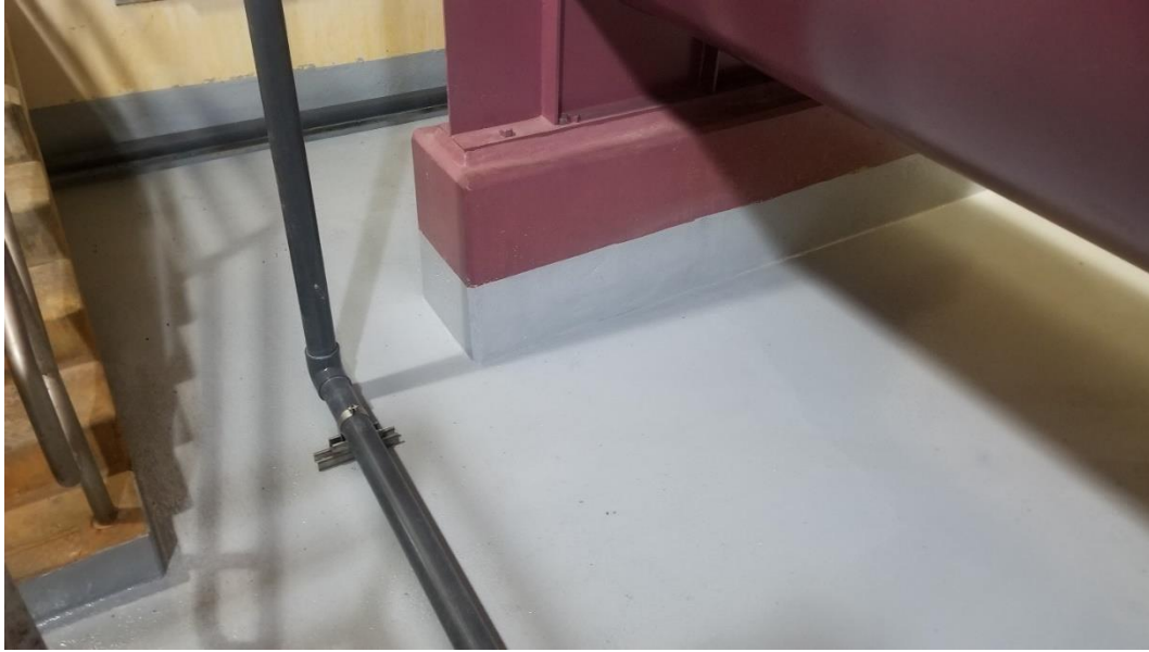
Repaired Concrete Support and New Containment Coating
