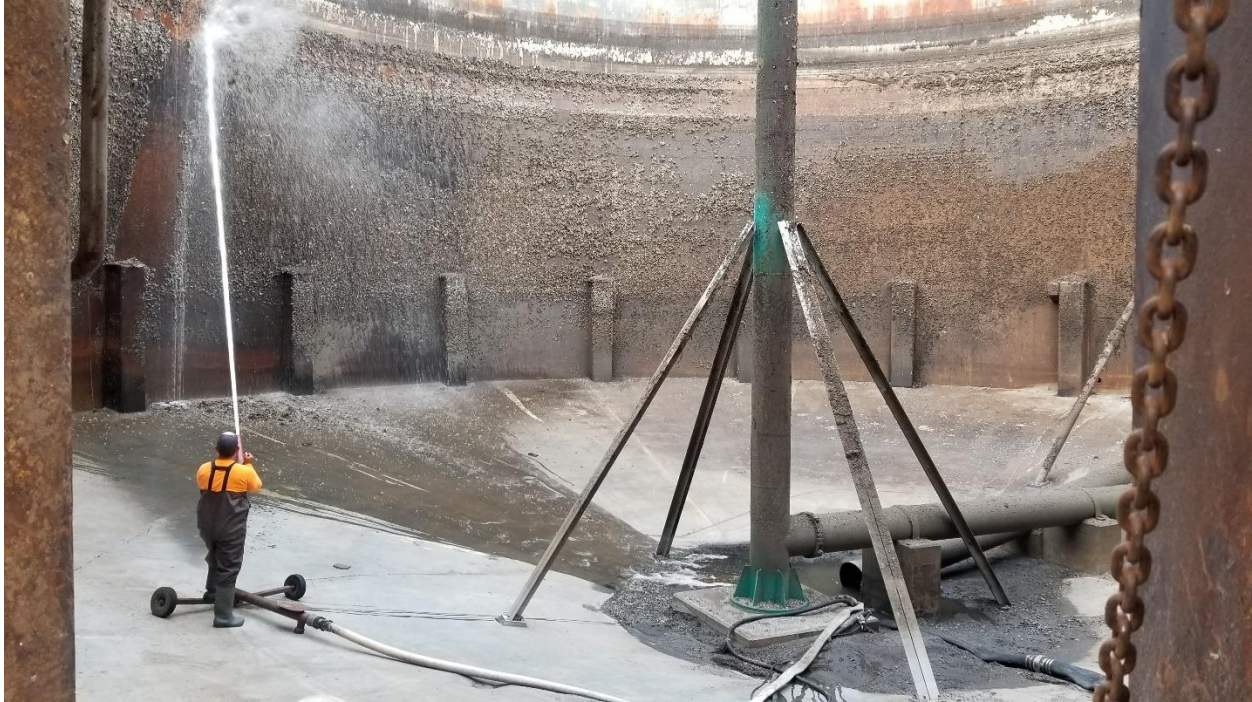
Inside Digester No. 2, cleaning of wall deposits in progress
