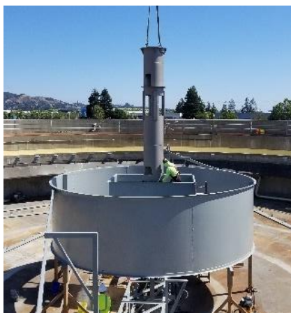
Installing new center column/RAS pipe.
