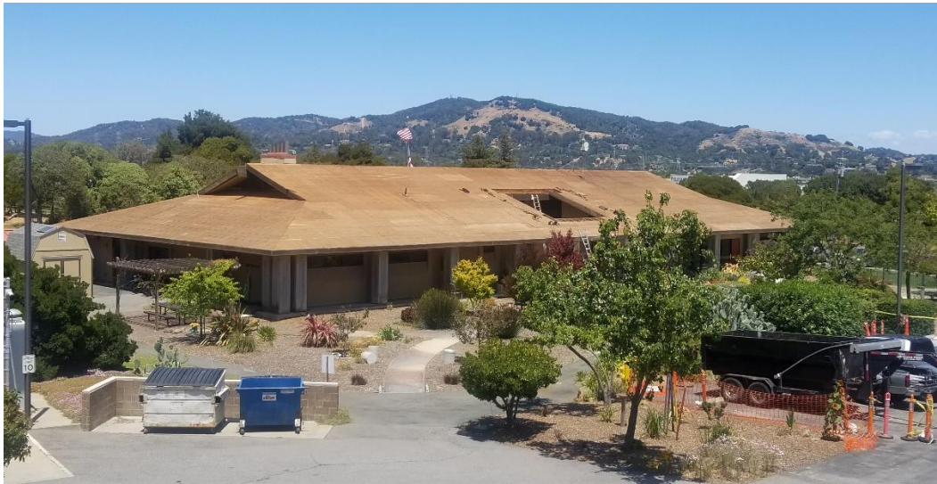
Demolition of underlayment, skylight framing and metal panels.
