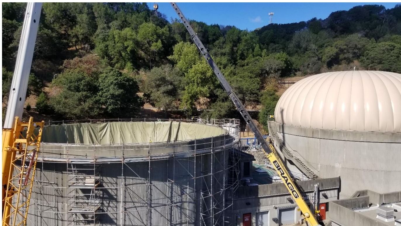
Digester No. 2 Cover Removal
