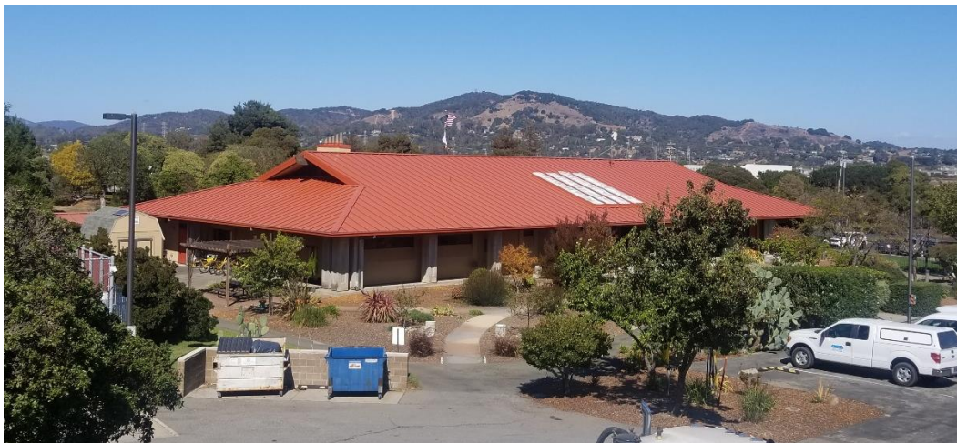
New metal panel roof and skylight framing.
