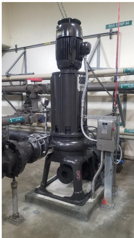
RAS Pump after replacement.
