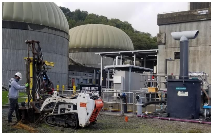
Above: Geotechnical boring for new above-grade storage tank location. Below: New Screening System
